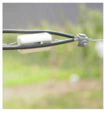
Gallagher Recommends – re-tightening joint clamps as part of a regular spring fence maintenance program.
