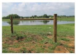
Although "H" braces afford optimum strength because they consist of two posts in the ground, it's not always easy to accomplish - especially if you're building in rocky soils. When just getting one post in the ground is a challenge, construct a "floating" brace.
