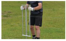
Tie off the top and bottom wires to the end strain insulators and any angle or corner insulators. Leave the tails long enough so they can be used for electrical connections later (see diagram on page 29). Next, tension the wires just enough to provide a straight line for positioning the line posts (see 4. on page 29).
