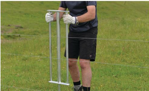
Tie off the top and bottom wires to the end strain insulators and any angle or corner insulators. Leave the tails long enough so they can be used for electrical connections later (see diagram on page 29). Next, tension the wires just enough to provide a straight line for positioning the line posts (see 4. on page 29).
